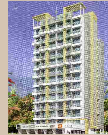
SILICON RESIDENCY ROADPALI, KHARGHAR
